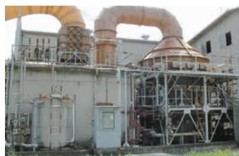
Gas emission washing treatment facility (Tokushima Plant (Kitajima location))
