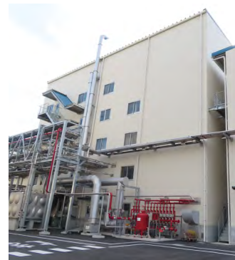
New insoluble sulfur plant
