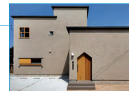
Exterior finishing materials
